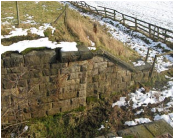
View of missing bridge which we suggest is in-filled, having first recovered the masonry to use on bridge repairs elsewhere along the line
