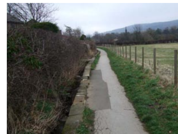
View to SE narrow width with fast flowing drainage channel. Between 0.5-1.0m extra width available to fence/hedge line for most of this section
