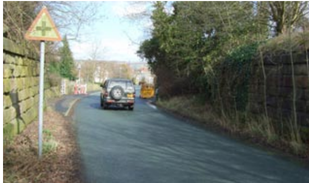
Menston Old Lane showing the substantial abutments left from the former bridge
