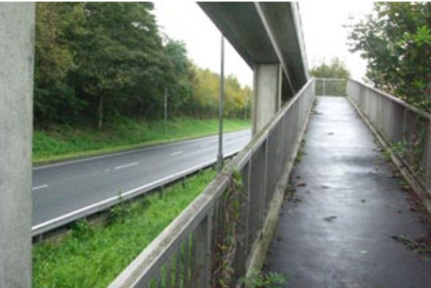
View looking up the zigzag ramp leading to the bridge over the A660. On the south side, the bridge runs into the lane up a short, well-graded ramp. The parapet heights are slightly low for cycle use at approx 1.2m and so we suggest that for the span over the road itself, it would be sensible to raise their height to 1.4m by clamping an extension onto the existing rails.
