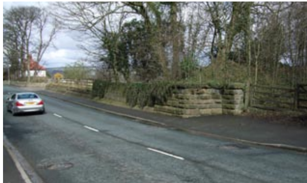
The remaining abutments of the Bradford Road Bridge which would form the basis of an embankment leading up to a new bridge crossing. The gates on the right would be the location of the works access
