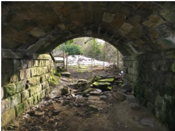
View under bridge. The public footpath runs through there, as does a twin slabbed water culvert. It would be desirable to tidy all this up and probably seal the surface to ensure no further damage from flood water
