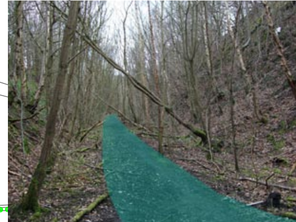
The railway path runs through a dramatic steep-sided 6m cutting. There are good opportunities for artwork and seating to overlook the neighbouring golf course just prior to this section. The tarmac path would be set on a low causeway to maintain drainage
