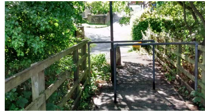
Figure 22. Staggered barriers south end of abovefootbridge
