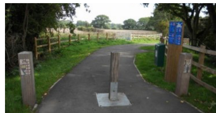
Figure 26. Example of single lockable bollard
